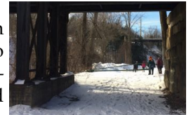
Proposed trail will pass under the RR trestle and Route 5 bridge in Bellows Falls.
